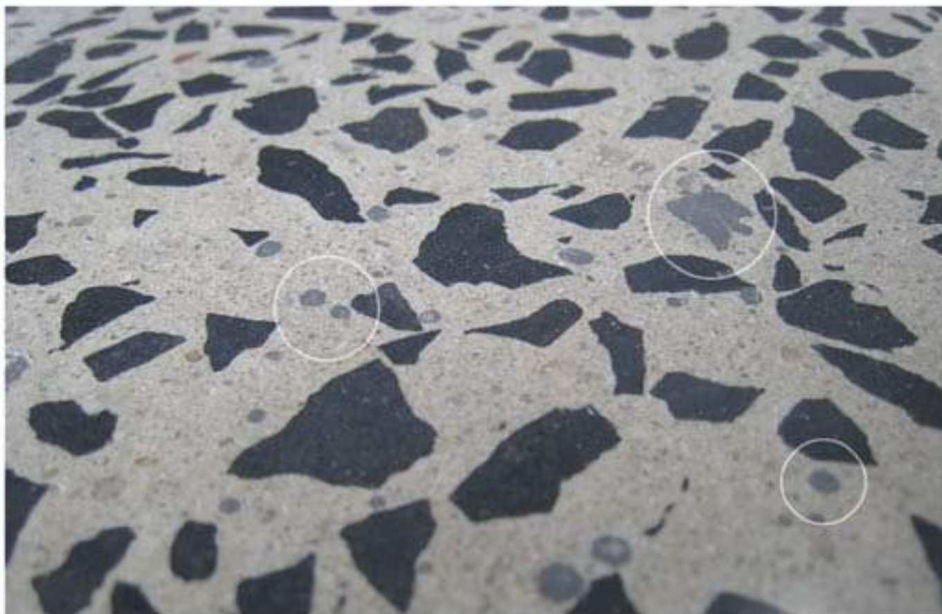
Holes filled when grinding with 120 grit metal-bonded diamonds and GM 3000™.
